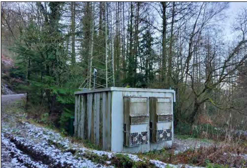
Figure 3-18 - Metal Building Connected to Tower
