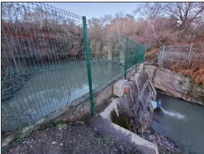
Figure 3-13 - Small Quarry Pond with Controlled Discharge
